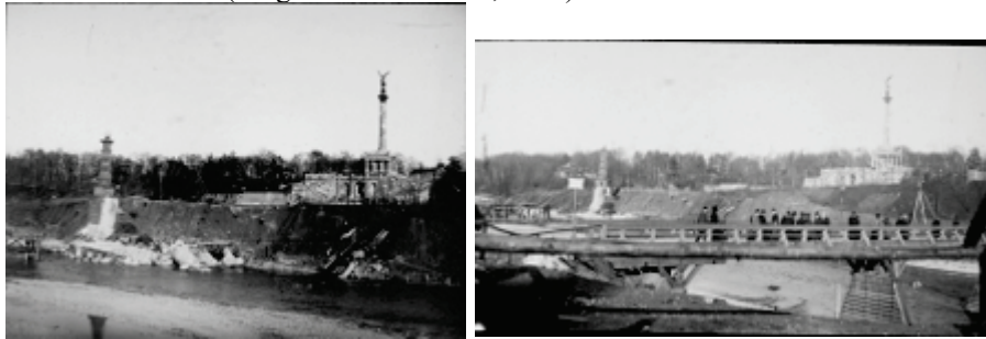
Fig. 3. Collapsed Luitpold bridge after the 1899 flood (left) and “emergency bridge” constructed as a temporary replacement (right). Both images were cropped to content. (Source: Wehrli, 1900a, 1900b).
